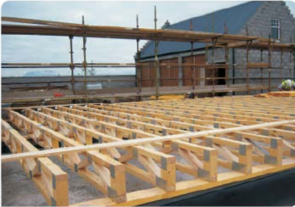
PICTURE : FloorTrus JOISTS ON ANOTHER OCHIL PROJECT
